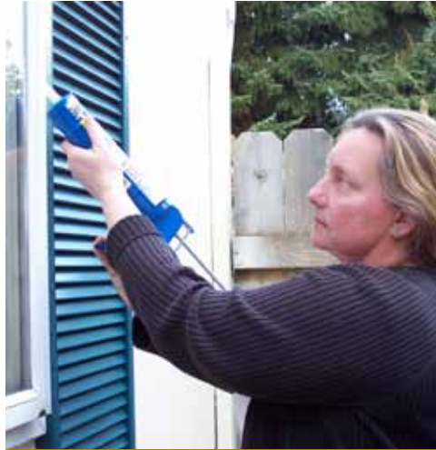
Mary McDowell cut heating costs by one-third after caulking her new doubled-paned windows and making other CEC improvements.
