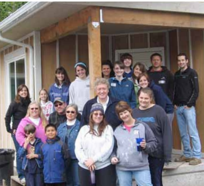
KulshanCLT Trustee and Habitat Women Build volunteer Shenandoah Myrick , in pink, and crew take a break from helping build a new home for Dawn Hubbard , front right
